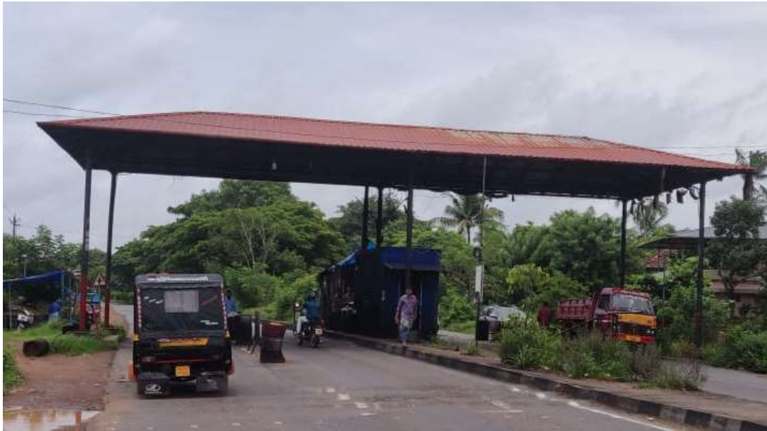
Figure 4-23 Muzhapilangad Toll Plaza
